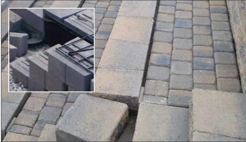
» The black sheet-like product placed behind the seat wall is a flat drain (12" tall x 3/4" thick) that BC Hardscapes used in place of the 6" drain tile used in the other bleachers. CL says, "It's a lot easier to install because you don't have to cut a trench in the middle of your gravel. You just put it on the back of your wall and put your gravel behind it. We'll watch to see which drainage method works out better over the years."
