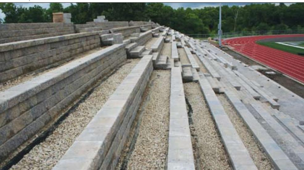
» The center of the bleachers is the highest point so water will drain in both directions. Most of the bleachers use 6" drain tile below each paved area which connects to larger drain tile and then underground storm sewers.
