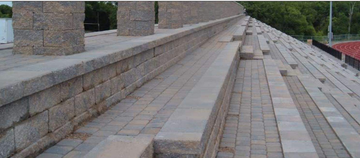
» The initial drainage design left every 10th paver space in the row against the seat walls back filled with 3/8 drainage rock. CL is developing plans to modify this before kids dig the gravel out.
