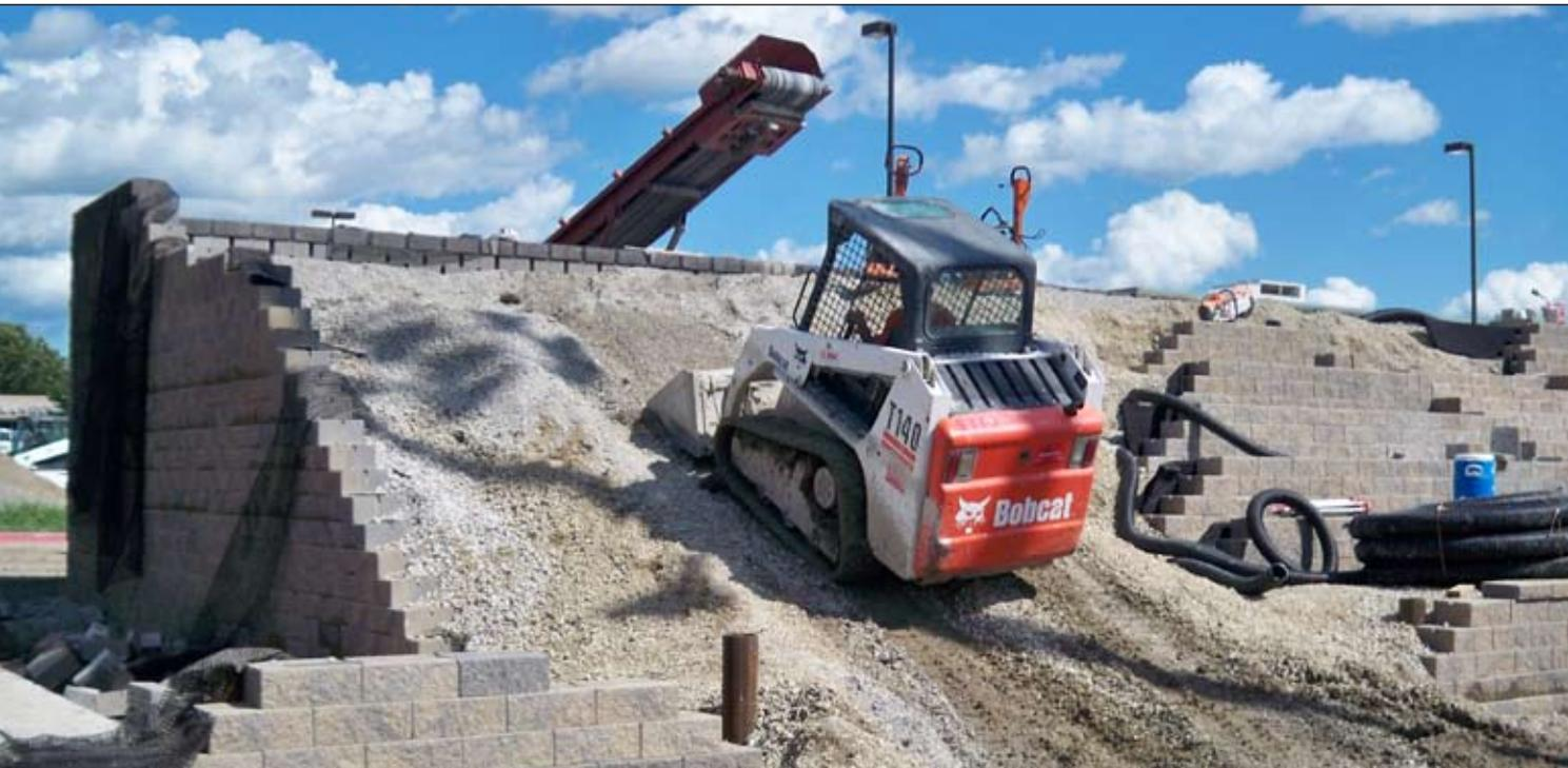
» Access was the biggest obstacle for BC Hardscapes in building the 4-wall bleachers (no side terraces). They left one end open so they could drive smaller equipment in. Earlier in the project, they kept open a larger access area that allowed them to drive dump trucks right in as they built the 16' back wall. Randy says they closed the larger access area off when the fill was about 8' high because it got too steep.
