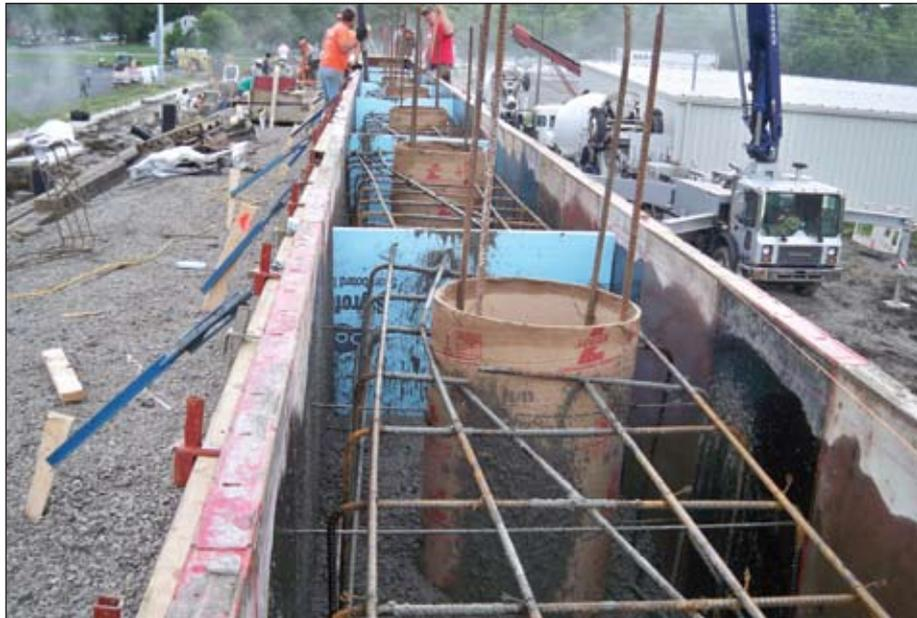
a 3' x 3' reinforced concrete grade beam that runs the length of the structure behind the last bleacher and the top 3' of the wall. Randy says, "We had to stop wall building to form the entire beam. We used concrete panel forms and brought a concrete pump truck in that pumped the concrete in."
