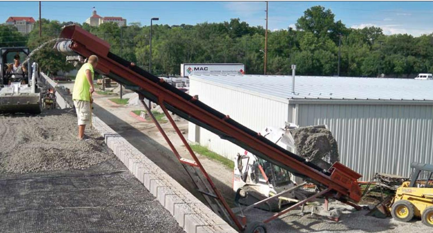
» When the back wall and backfill area was 8' tall and too steep to drive in dump trucks, BC Hardscapes began using their 50' conveyor to deliver gravel over the back wall. The conveyor is run off skid-steer hydraulics. The skid steer also tows the conveyor around the site.
